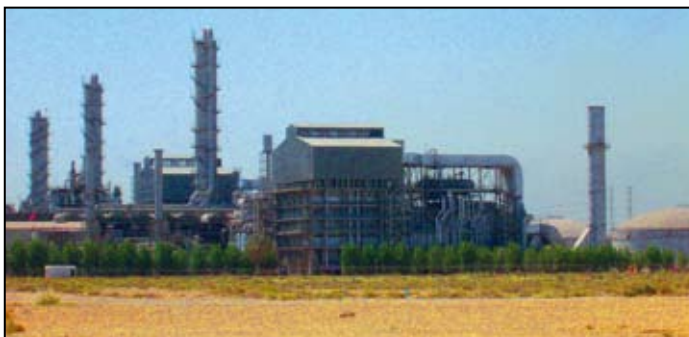
FIGURE 1. This photo shows the methanol production facility of Arrazi in Saudi Arabia
