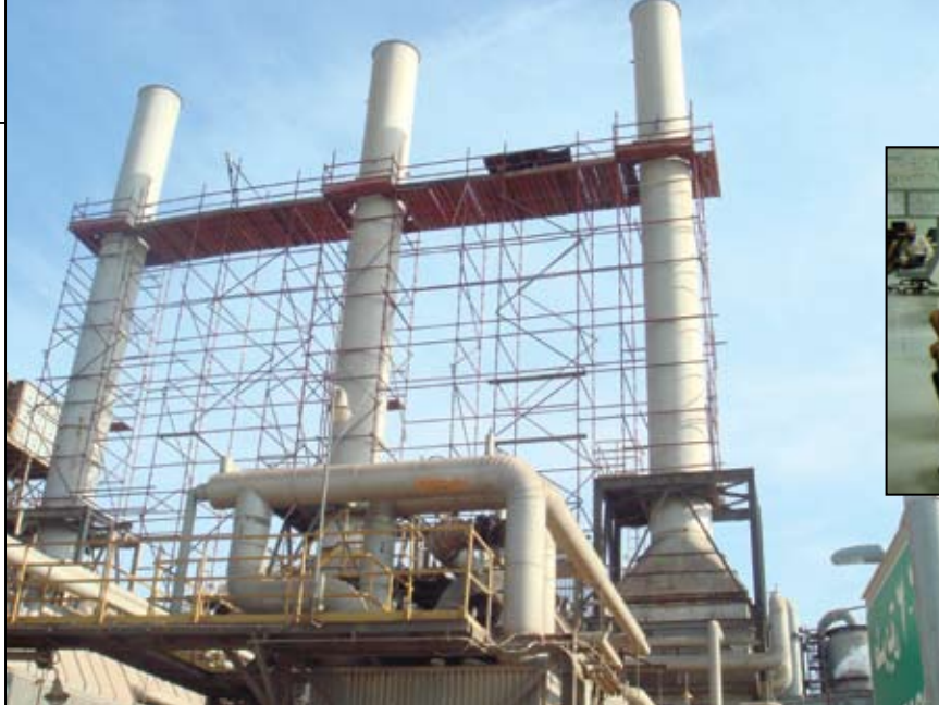
FIGURE 2. PEMS was implemented on the boiler stacks at Arrazi, three of which are shown here
